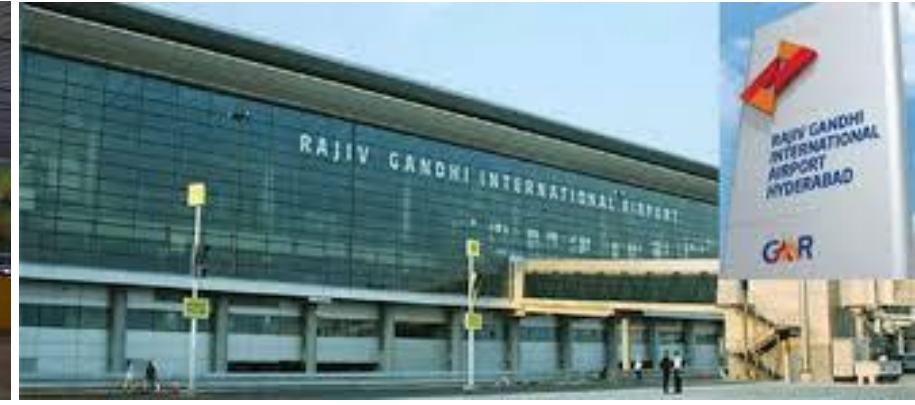
Good thermal insulation properties @ Terminal glass Façade: U-value = 1.4 W/m 2 K, SC =0.47
